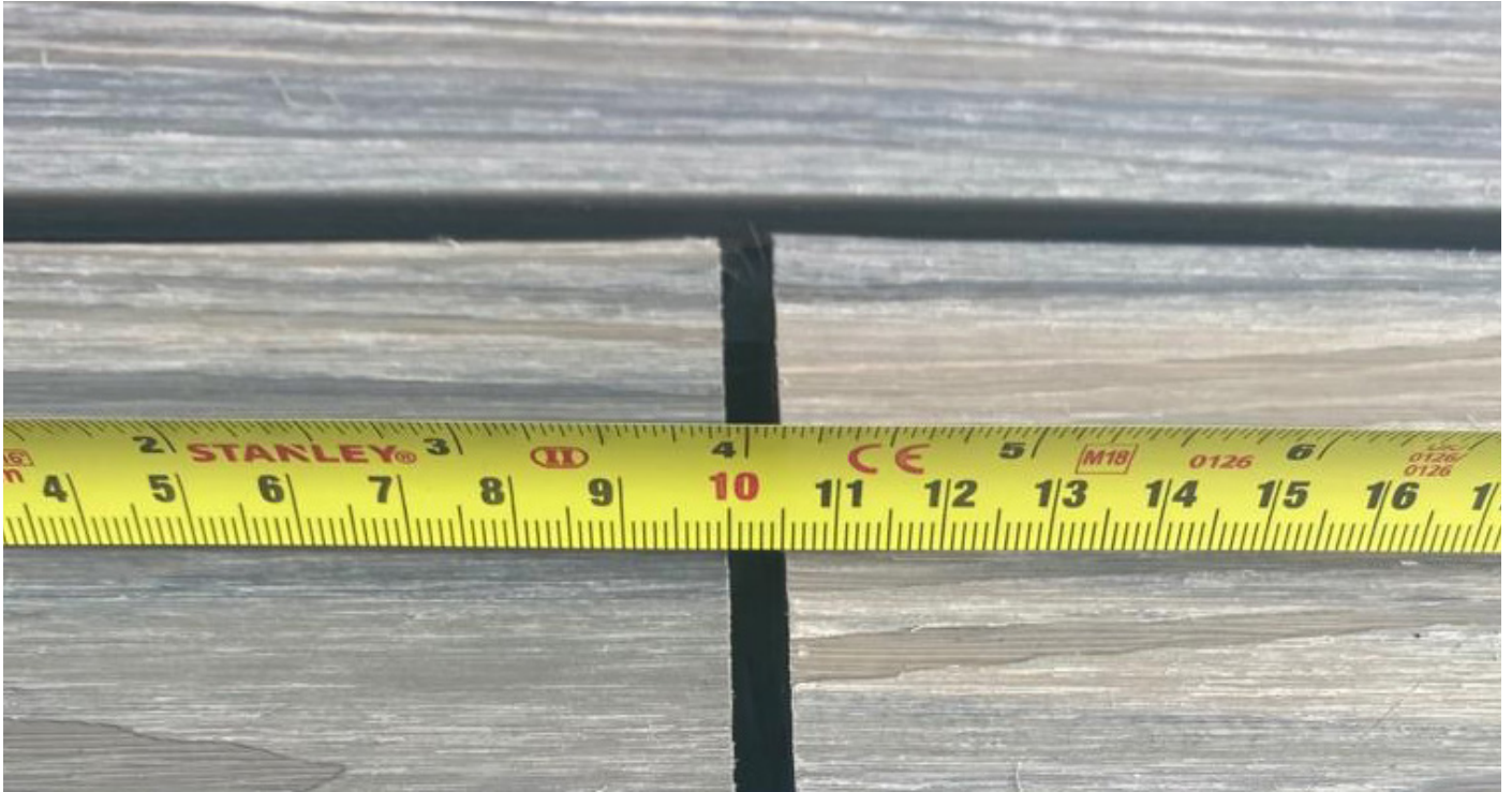
Expansion Gaps at Board Ends
